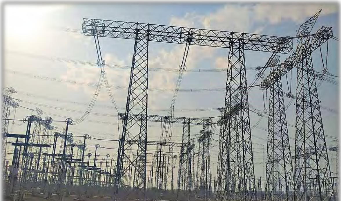
2x1500 MVA, 765/400kV Warora Substation
